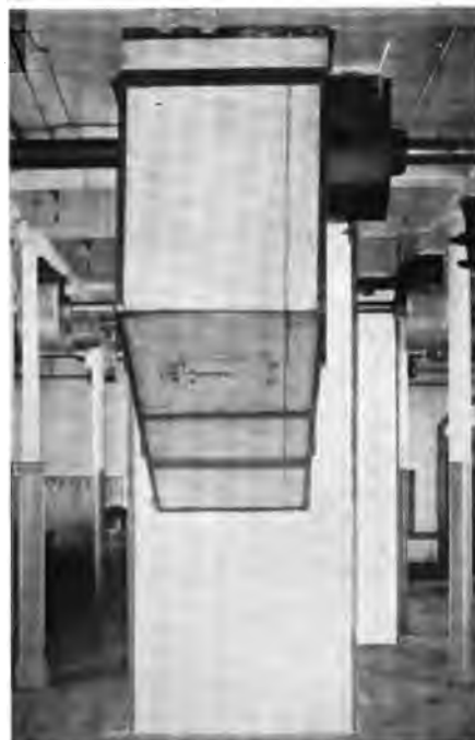
Fig. 4. Fire-Resisting Belt Enclosure.‡
